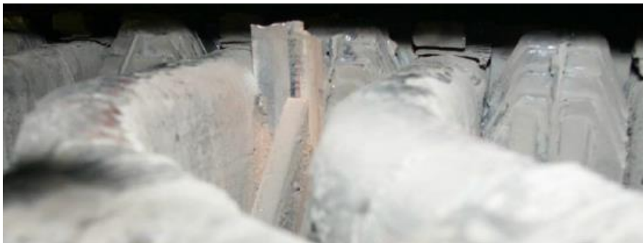
Figure 11: View from boroscope inspection. Image source: JIP project.
