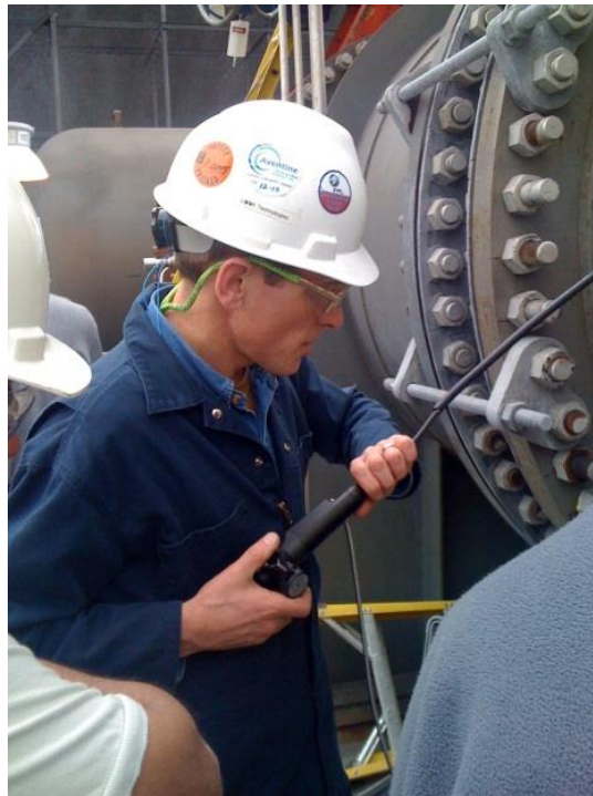
Figure 9: Boroscope inspection. Image source: JIP project.
