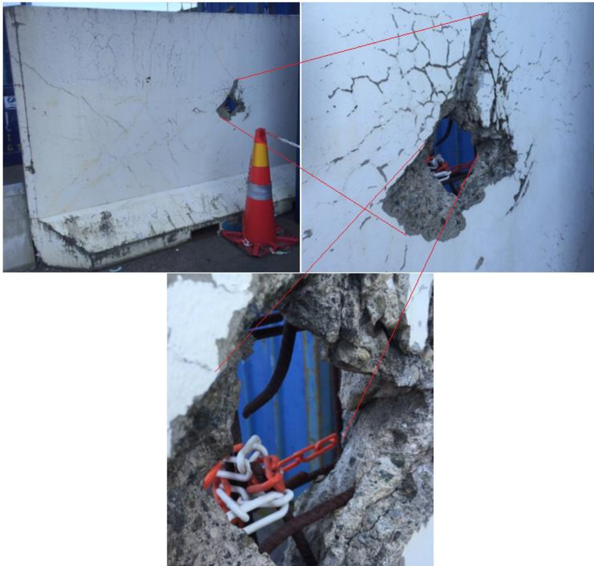
Figure 12 Penetration of safety walls
