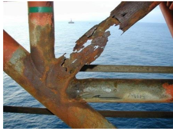
(B) Corrosion
