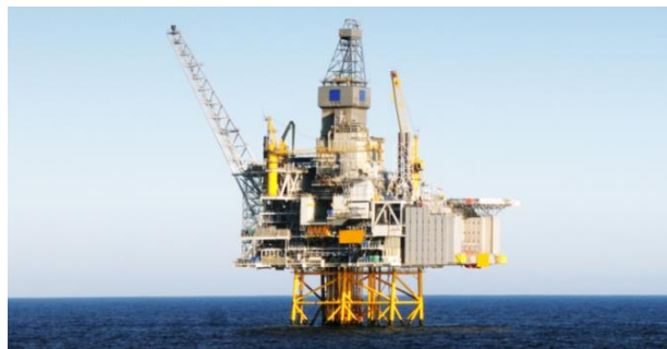
FIGURE 1-1: OFFSHORE JACKET
