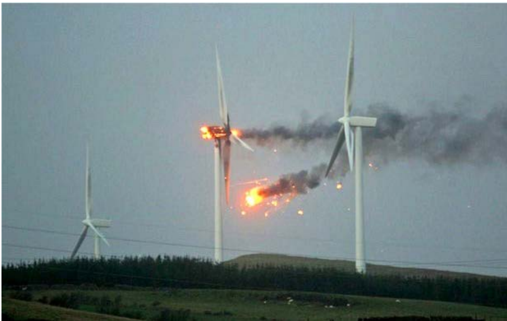
Figure 3: Fire at the Ardrossan Wind Farm (Telegraph 2011)
