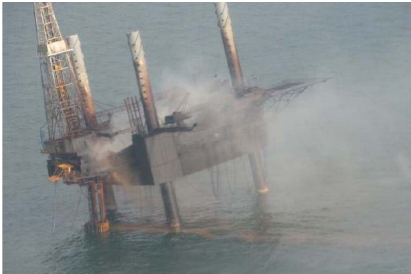
Figure 12: Usumacinta Jack-up Leaning Against Kab-101 Platform (Versatel 2007)
