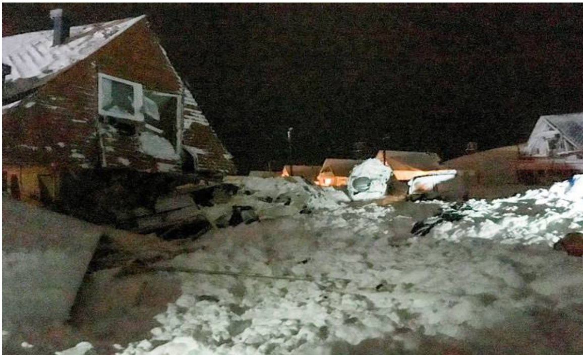
Figure 2.8: Damaged houses by snow avalanche in Longyearbyen, Norway (Newsdesk, 2015)
