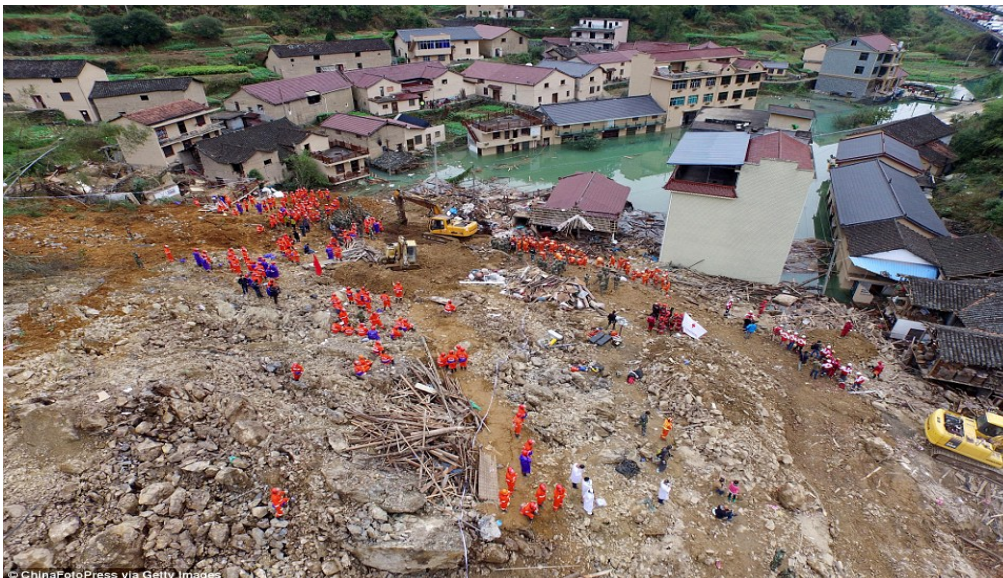
Figure 2.2: More rainfall resulting flood in the Lidong village after landslide (Lyne, 2015)
