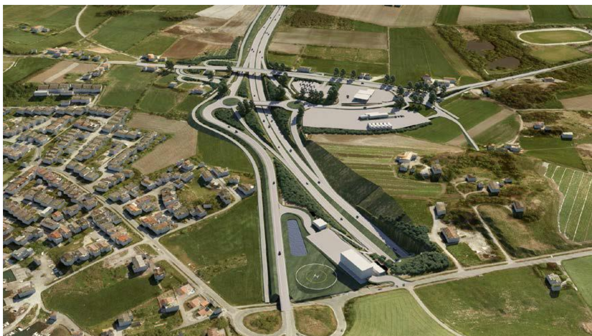
Figur 2: Tunnelmunning Harestad (Statens vegvesen, 2016)
