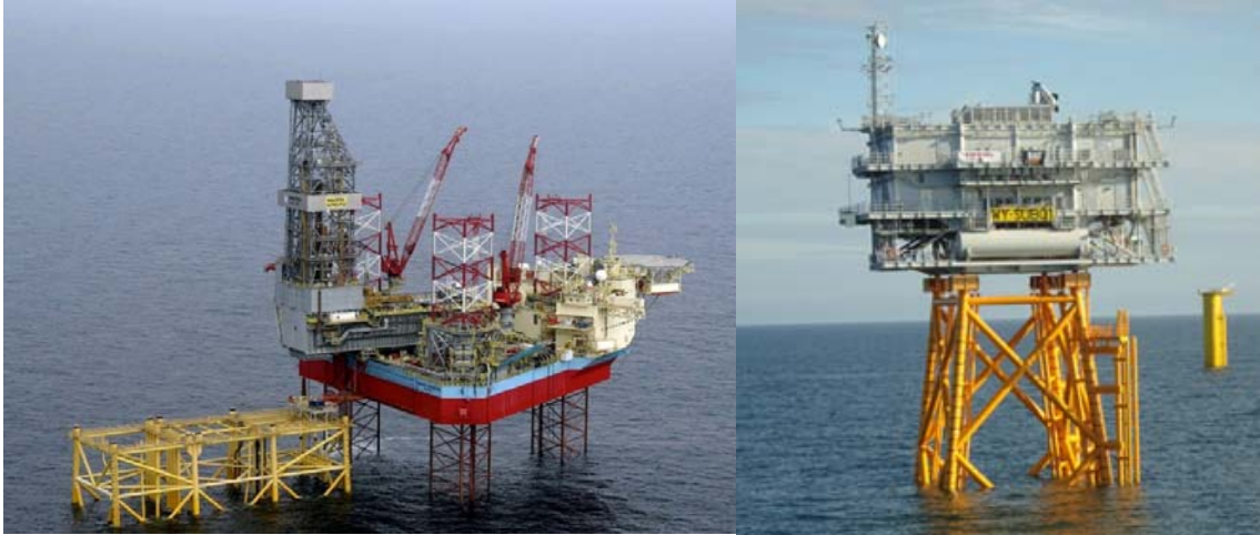
Figure 7 Jack-up rig predrilling on a jacket. The jacket is the yellow construction Figure 8 Topside installed on a jacket
