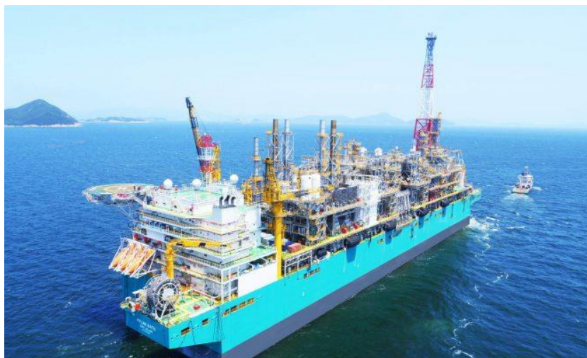
Figure 6.4 First Operating FLNG in the World: PETRONAS FLNG Satu in Kanowit Gas Field, Malaysia Figure Source: PETRONAS (2017a)
