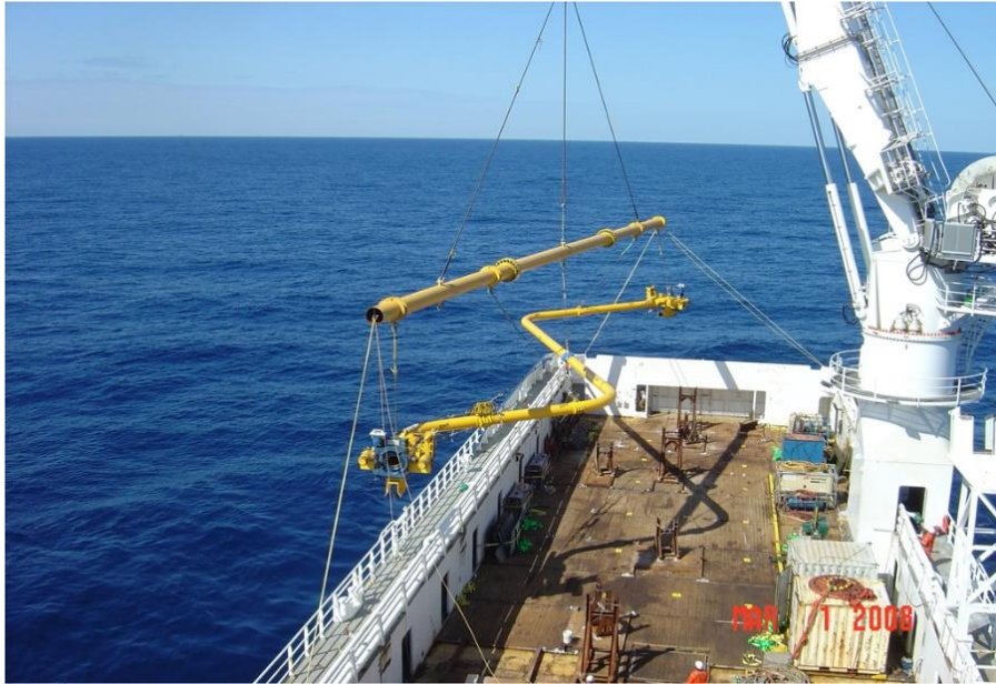
Figure 2.2. Rigid spool (Spool, 2008).
