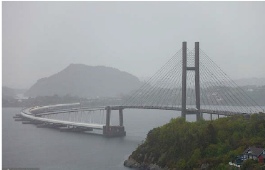
Figure 1-3 An existing floating bridge: the Nordhordlandsbru near Bergen. The nearest span constructed as a suspended bridge to enable ship traffic. Ellevset (2011).
