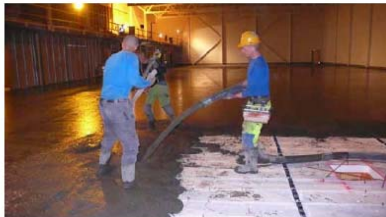
Photo 1: Casting of 'Mapecrete System' floor 1300 m 2 jointless.
