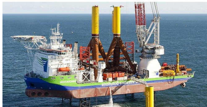
Figure 1.5 Tripod installation by jack-up vessel (Overdick GmbH & Co KG, 2012)
