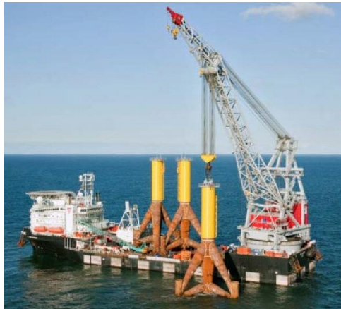
Figure 1.4 Tripod installation by HLV (HeavyLiftSpecialist, 2013)
