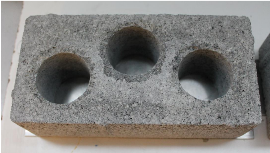
Drilled holes in a concrete block (FCC-1)
