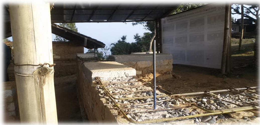
Mode structure with earthquake resistant RC banding (Photo: Mikael Johnsen)
