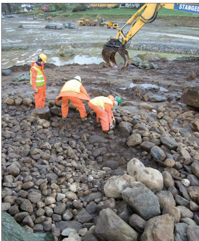
Figur 8. Stage 7, removal of the monumental stone mound with a digging machine provided with claws.
