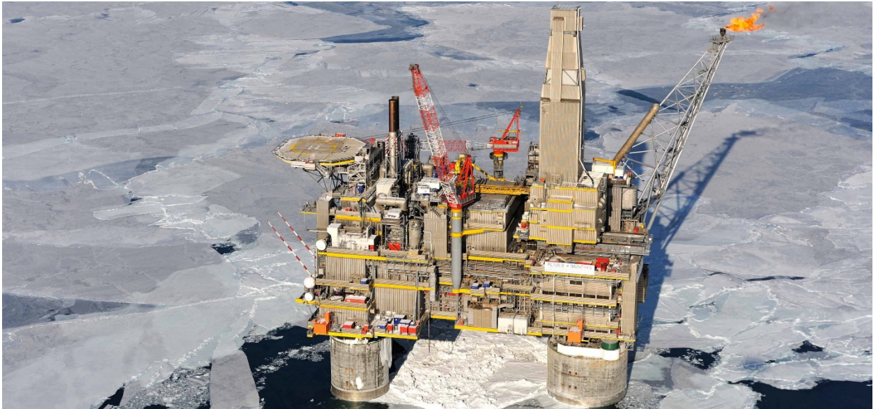
Figure 2-3. Piltun-Astokhskoye-B ( Sakhalin Energy, n.d. )
