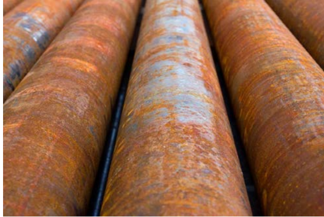
Figure 2.5: Example of uniform corrosion on pipelines [87]
