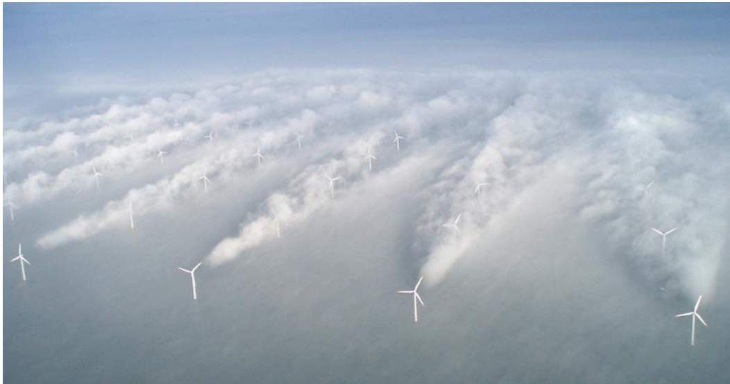
Figure 7 wake created by turbines. (Carbon-Trust, 2017).
