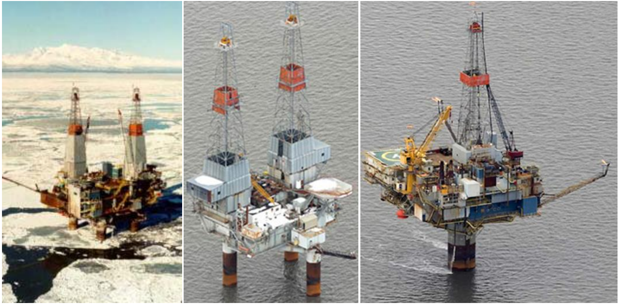
Figure 23: Offshore platforms of three possible configurations in Cook Inlet (Dolly Varden platform, Spurr platform, Monopod platform)
