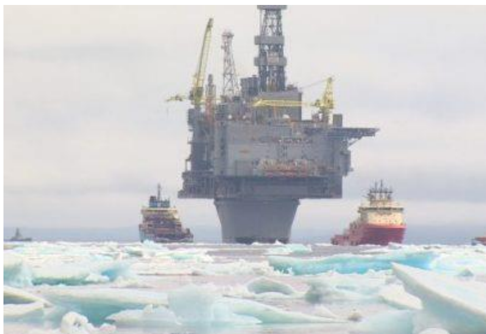
Figure 21: Hebron platform being towed-out to the field ( Hebron Project official webpage, n.d. )
