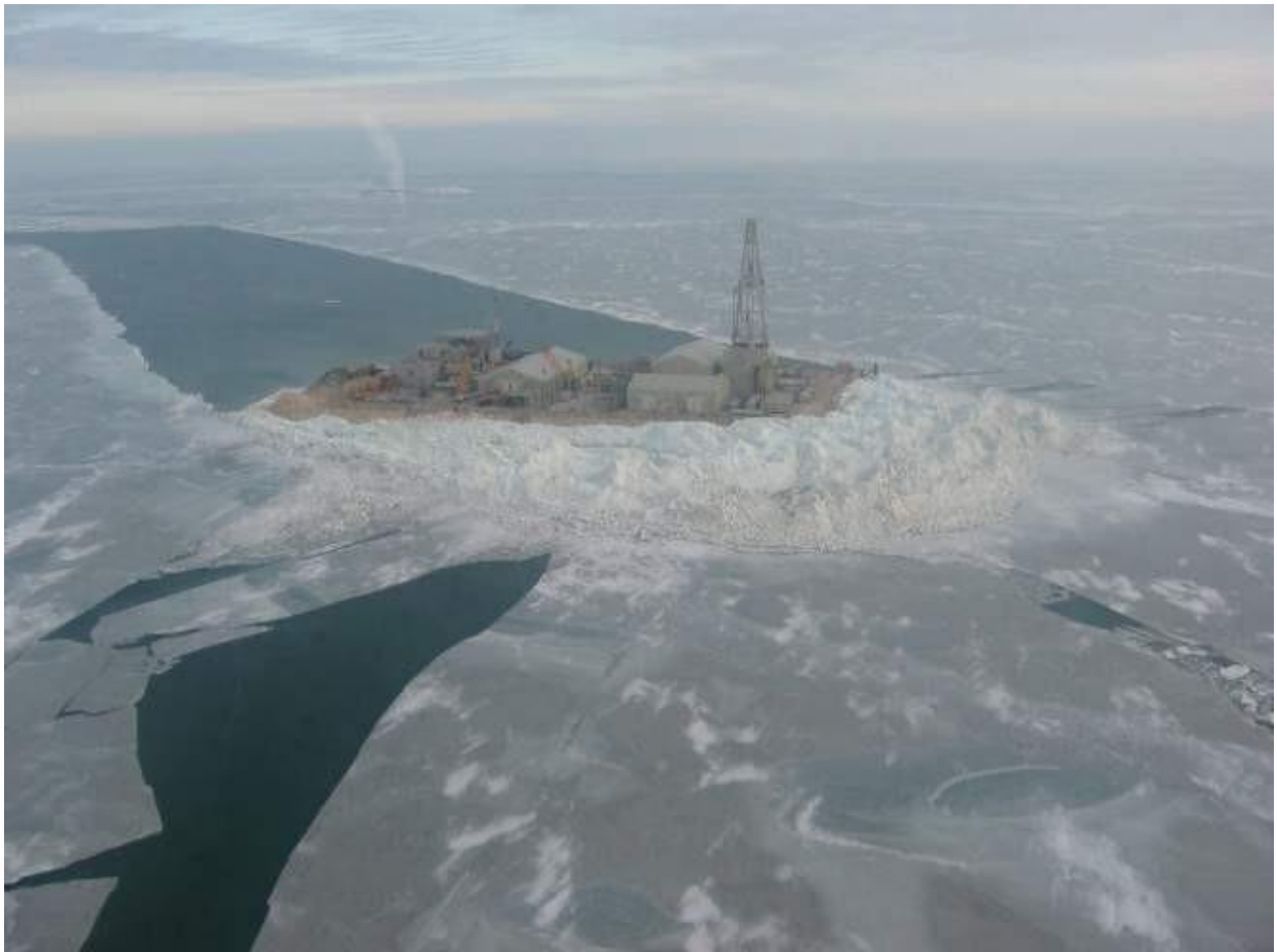
Figure 4.4: The Picture of D Island (Kashagan) wherein an ice wake can be observed behind the structure (Topaz Energy and Marine, 2015)
