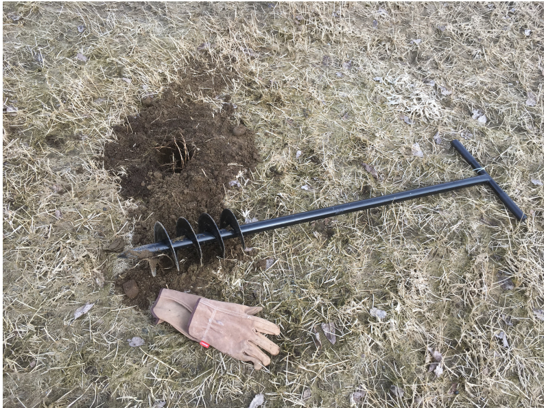
Figure 13: Geophone grounding preparation.
