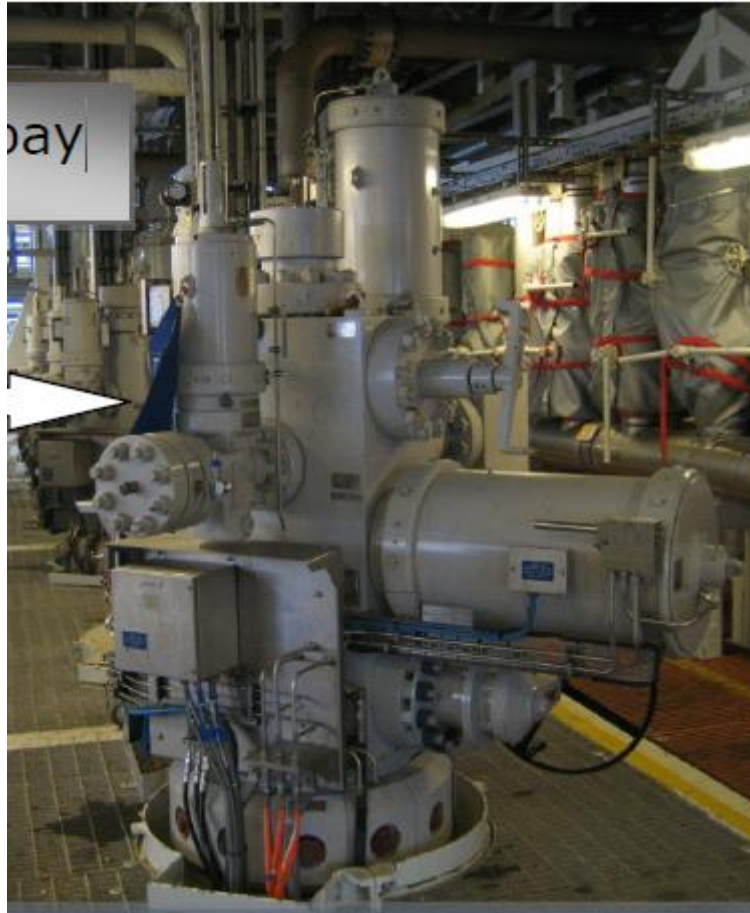
Figure 39: Platform well X-mas tree
