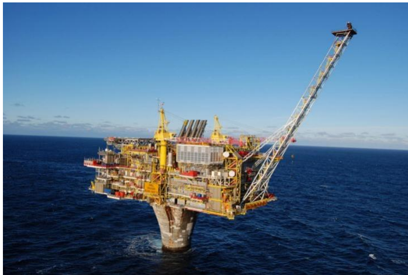
Figure 70: Draugen concrete gravity-based platform [208]
