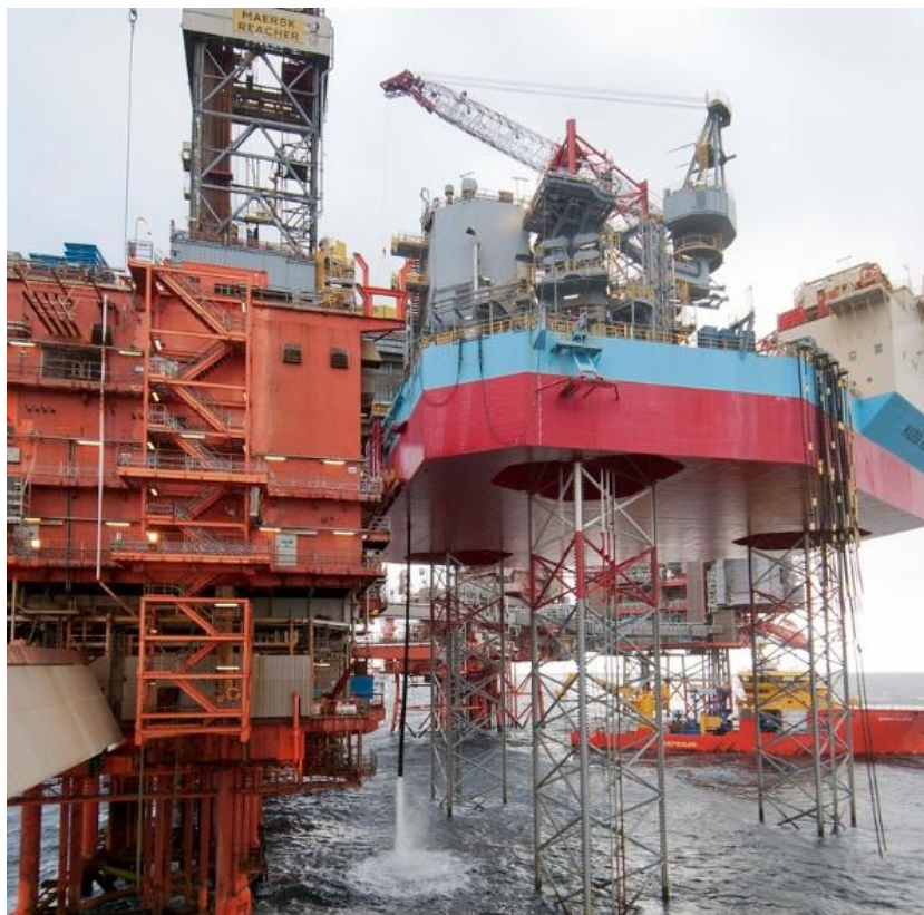
Figure 42: Maersk Reacher jack-up performing P&A on Valhall DP [110]
