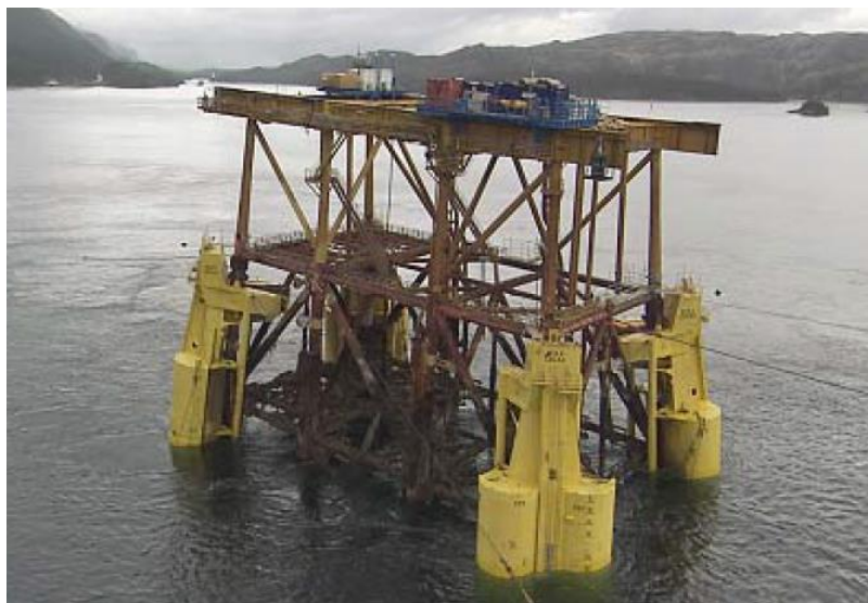
Figure 12: Flotation and removal of Frigg DP-2 jacket [25]
