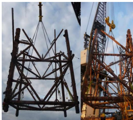
Figure 23: Transferral of the H7 jacket to land [51]
