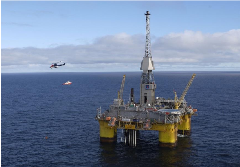
Figure 15: Visund A: a semi-submersible style production platform [28]
