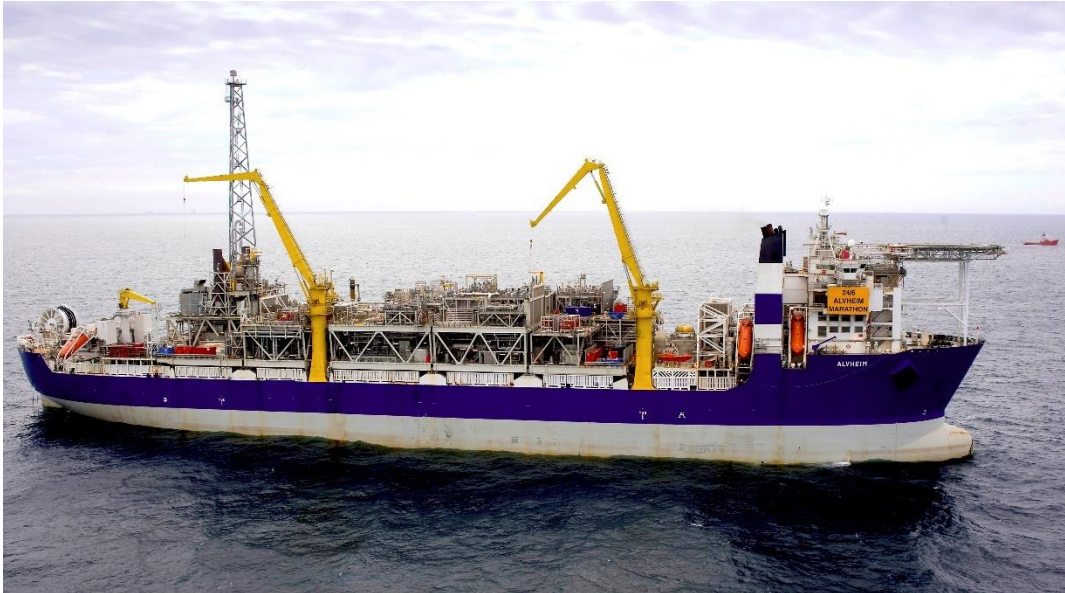
Figure 13: The Alvheim FPSO, a typical hull-shaped FPSO [26]
