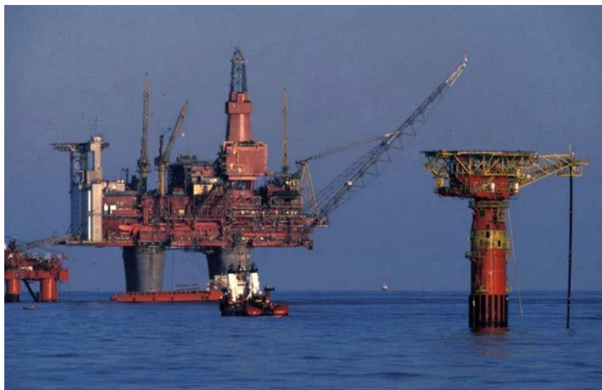
Figure 72: Statfjord C with the loading system in the foreground [210]
