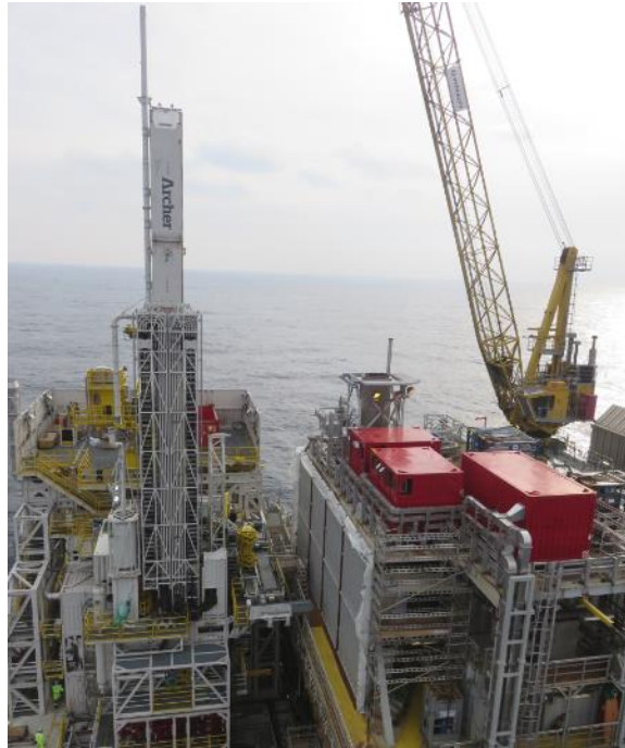
Figure 7: Archer MDR installed on the Heimdal platform [17]
