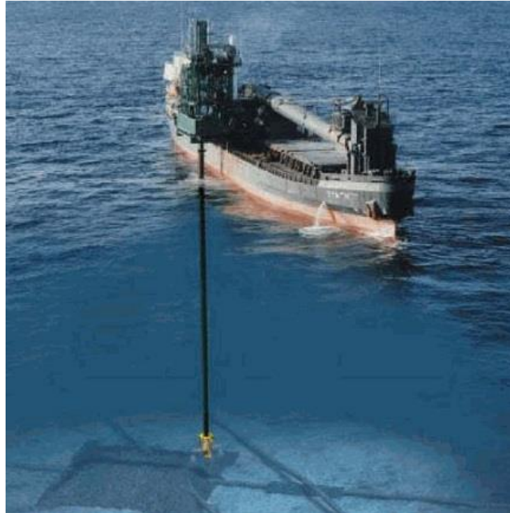
Figure 49: Rockdumping of pipeline
