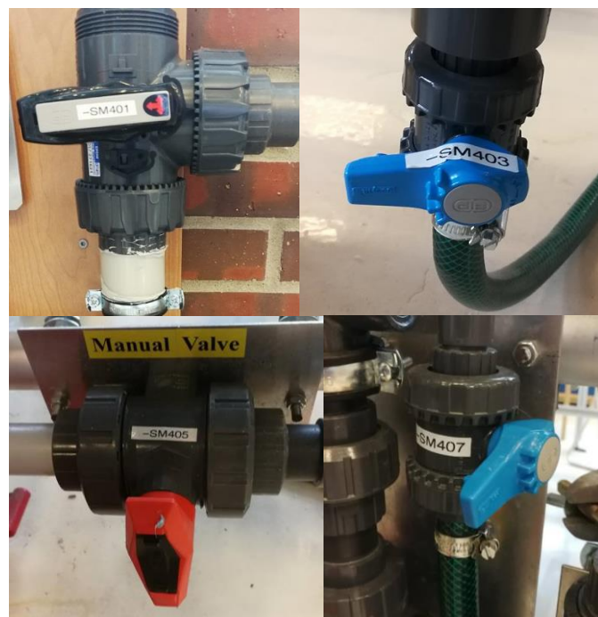
Figure 13 Correct position for valves in flow position
