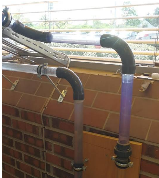
Figure 41 New setup for bend near pump output
