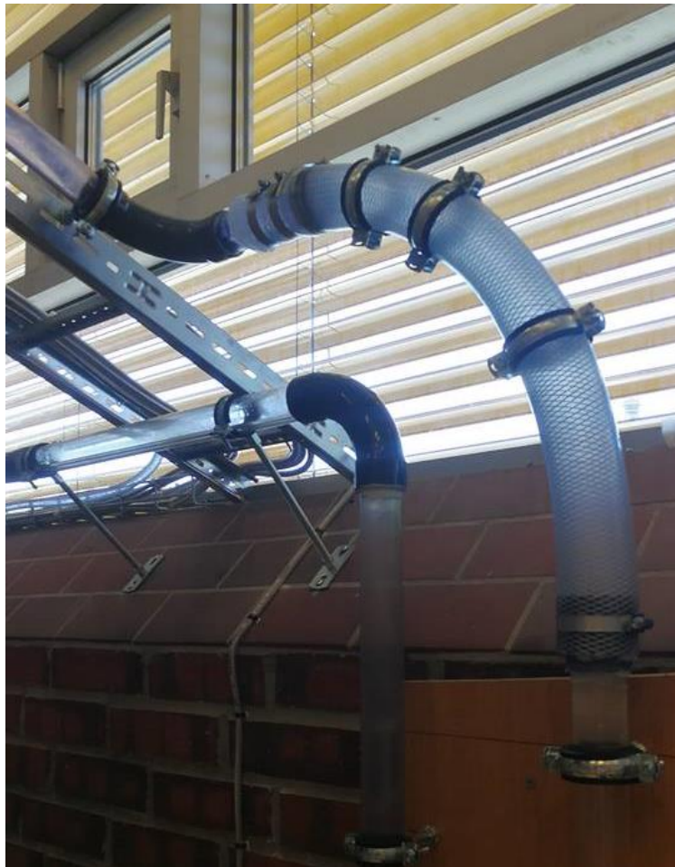
Figure 39 New pipe for leakage #2
