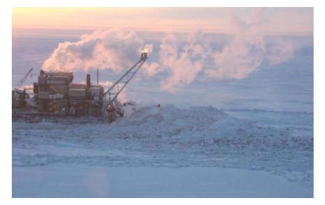
Figure 10 14.3-m Pile-Up on Northstar Production Island in Late January 2008 (60- 90 cm thick ice blocks encroached 27 m onto concrete mat during 30- to 40kt westerly storm; Coastal Frontiers, 2012)
