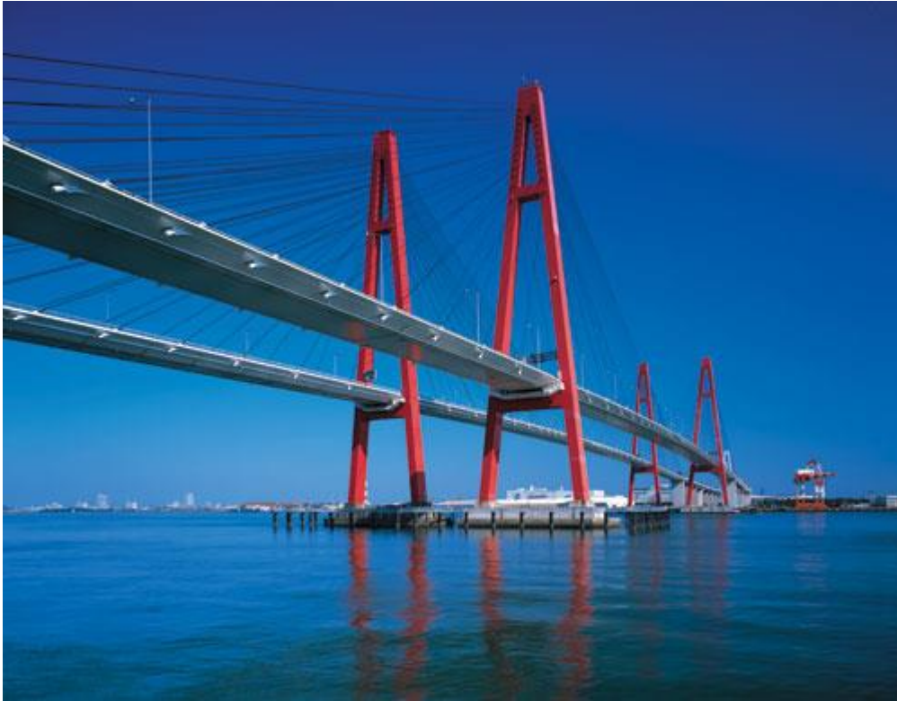
Figure 4.2 Meikonishi Bridge in Japan
