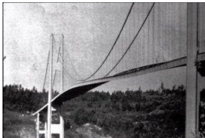
Figure 1.1 Flutter of Tacoma Narrows Bridge
