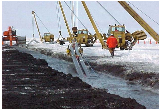
Figure 3.4. «Northstar» Pipeline Installation [7]
