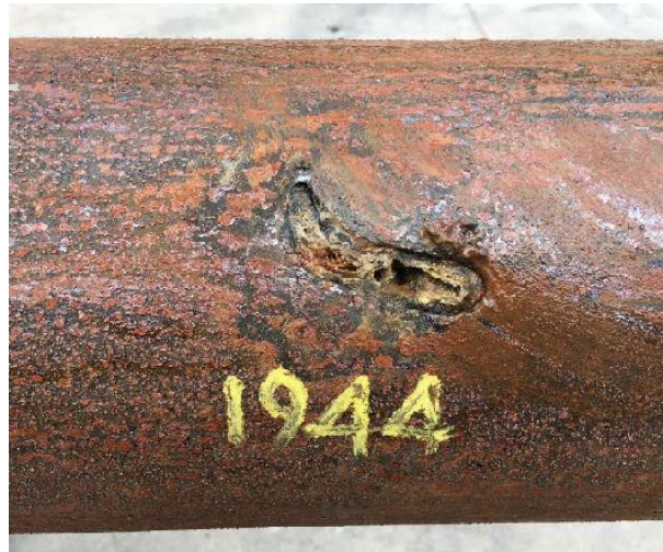
Figure 6.9: Heater burn-through resulting from burning a thermite mixture generating excessive temperatures. [Price and Elizondo, 2018]
