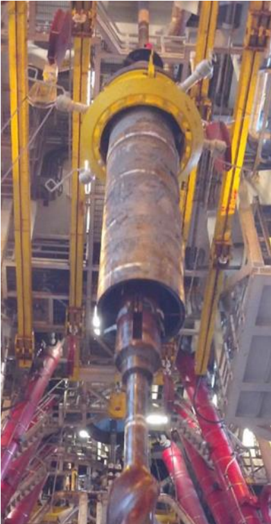
Figure 22 - Photo of UWR and cut wellhead. Source BHGE
