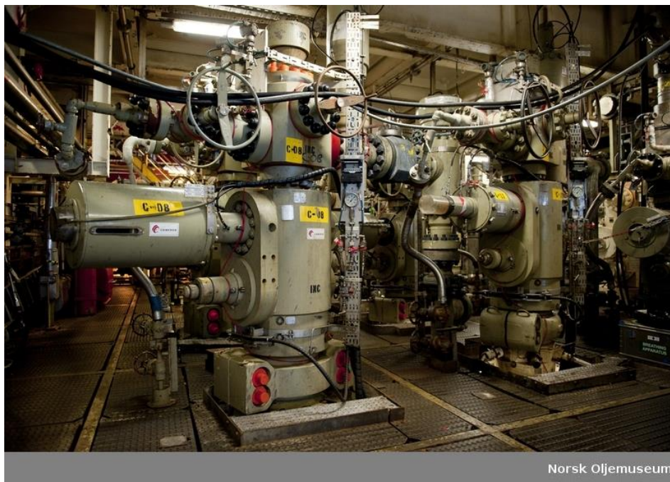
Figure 14 - Surface wellhead located on Statfjord C
