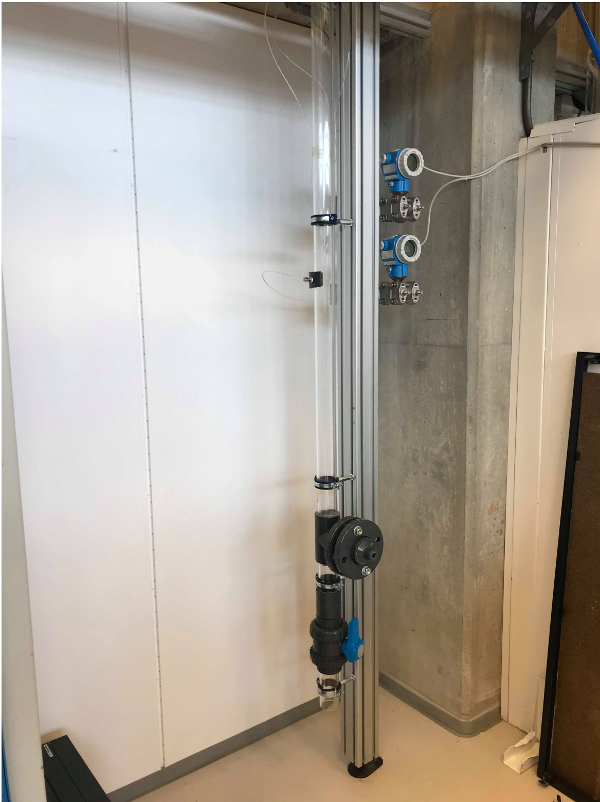
Figure 4. 8 Pressure inlet and gate valve to open and close the pipe
