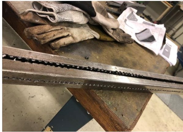
Picture 34. Optical box frames during construction.
