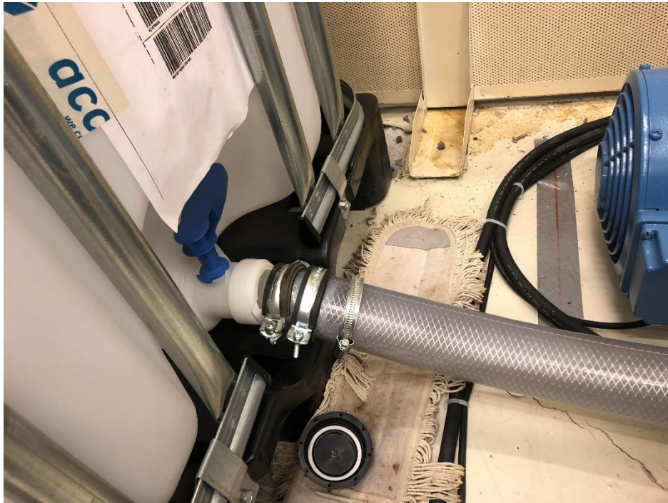
Picture 4. Tanks old outlets.
