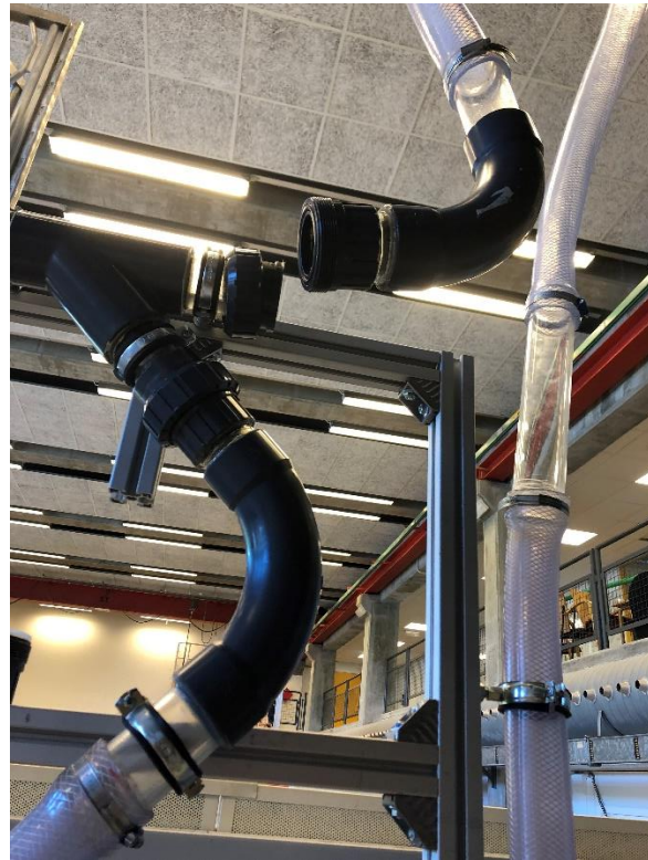
Picture 15. Mixing unit entry U joint.
