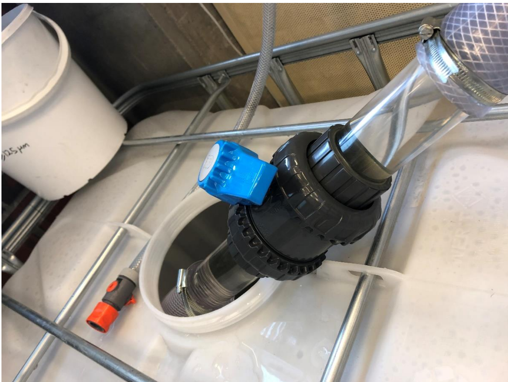
Picture 47. Separator outlet valve.
