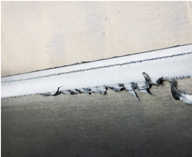
Figure 3-15 Defect at the frontside
