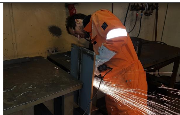
(h) Disassembly of strongbacks after the plates have cooled to 20 °C.
