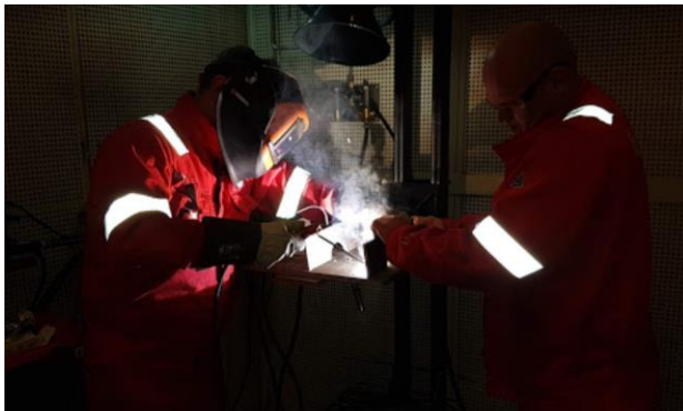
(g) Installation of strongbacks
