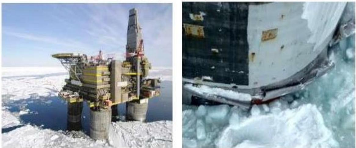
**Figure 2.5** Damage to the metal cladding on the supports "PA-B" [13]
