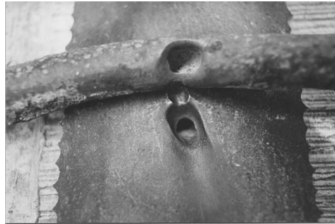
Figure 2.7: Pits in a galvanized water pipe that triggered the 1992 explosion of Guadalajara: corrosion of the gas line and the resulting leakage in a sewer main(5).
