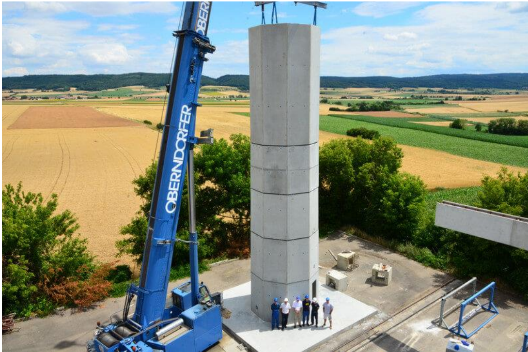
Figure 7 - Precast concrete tower during installation phase (Dvorak, 2016)
