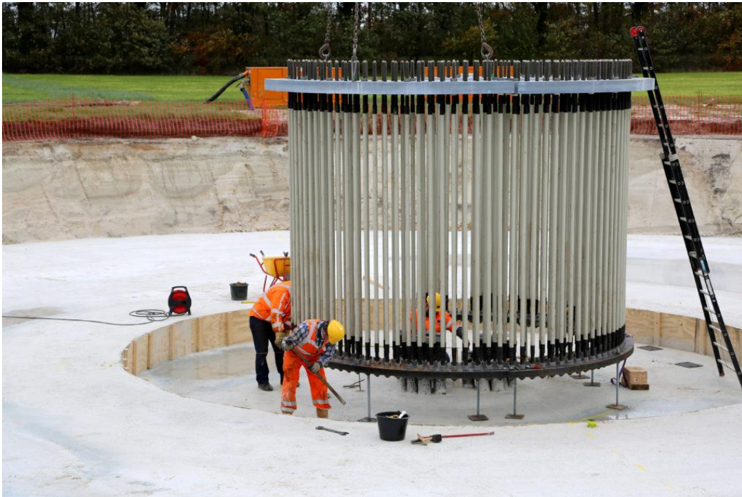
Figure 10 - Anchorage cage during the installation phase (CTE Wind International, 2020)
