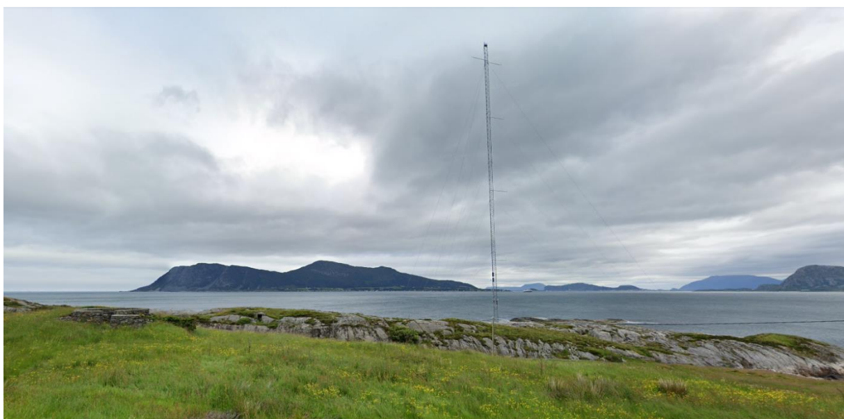
Figure 23 - The measuring tower at Kvitneset (Google Maps, 2020).
