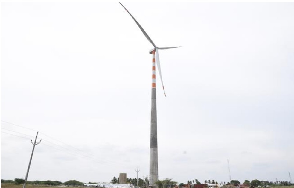
Figure 8 - Hybrid concrete and steel turbine tower (Financial Express, 2018)
