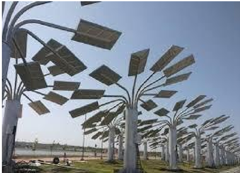
Figure 35 Solar Trees (Twitter Photo)
