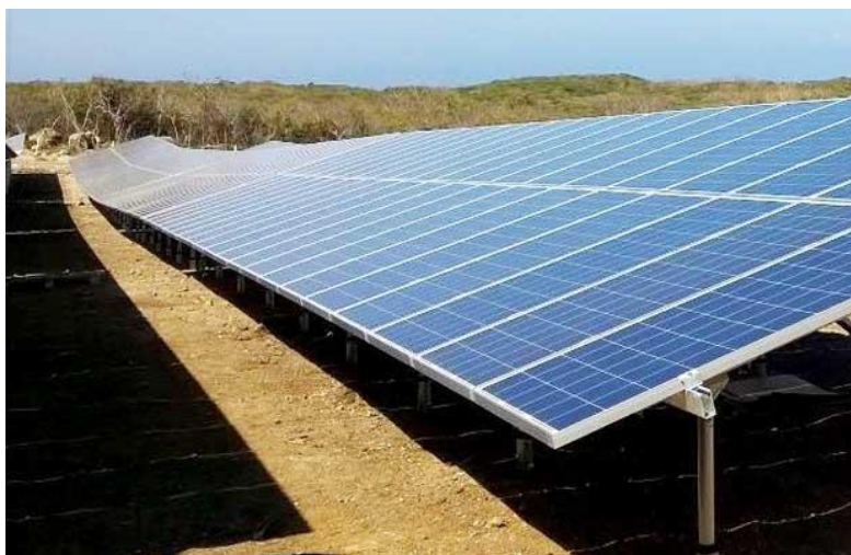
Figure 18 Solar Panel Inclination of 20 degrees at a solar power plant (google image)
