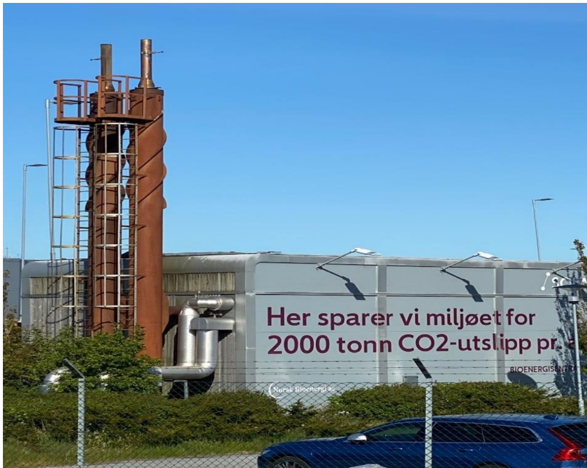
Figure 30 light black smoke observed from the chimney of the wood-burning plant that indicates particles
