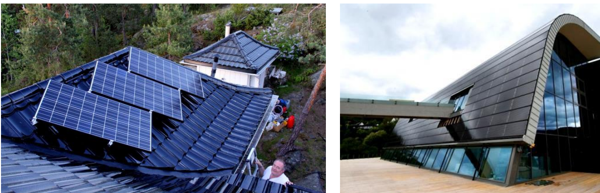
Figure 2-5- application of BIPV and BAPV systems, Roof-mounted BAPV, Chiko Solar, Norway (right); BIPV on the facade of Oseana Art and Culture Center, Bergen, (BIPVNO, 2019)
