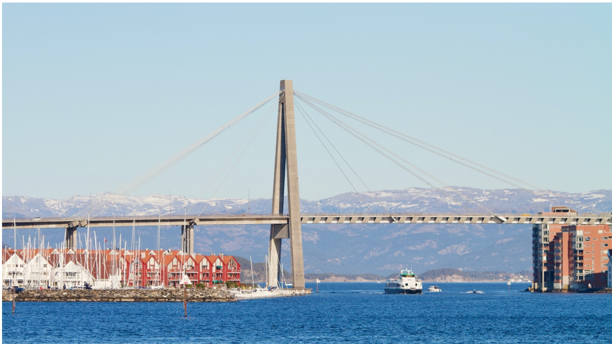
Figure 1: The City Bridge / Bybrua, Stavanger
