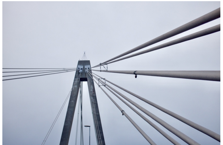
Figure 2: Stay cables of bybrua, North side of tower
