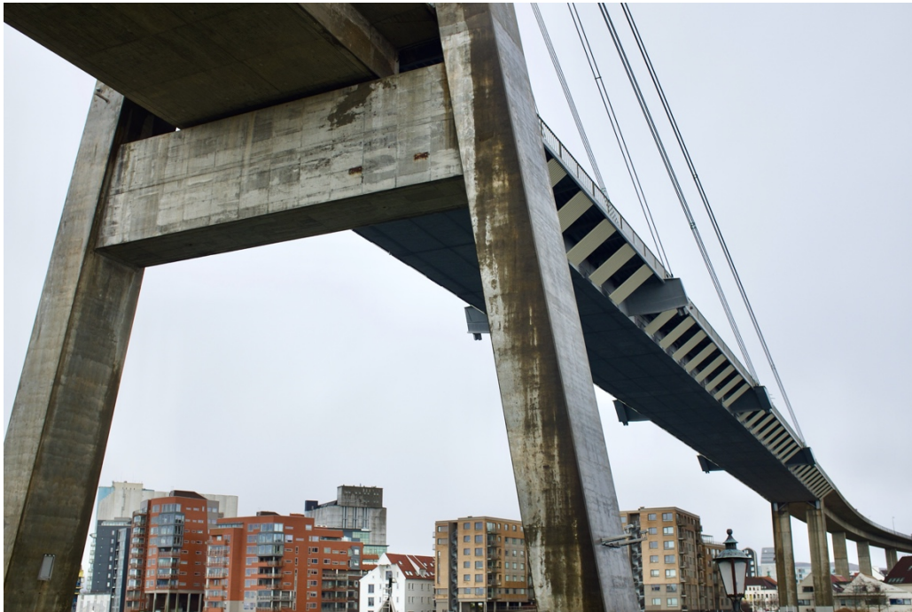
Figure 7: Main span of bridge, seen from underneath
