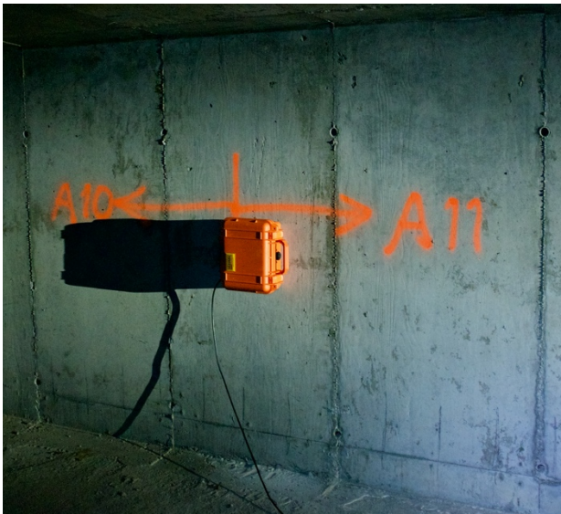
Figure 19: Accelerometer within concrete deck, between axis 10 and axis 11
