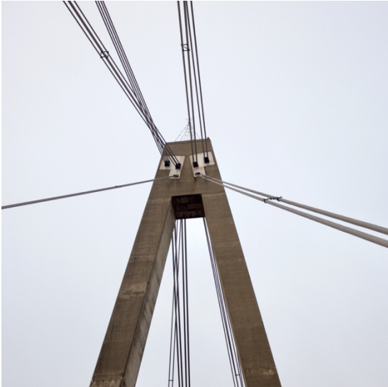
Figure 11: Top of tower
