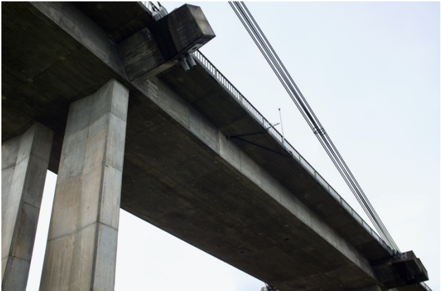
Figure 12: Crossbeams for anchoring at concrete deck
