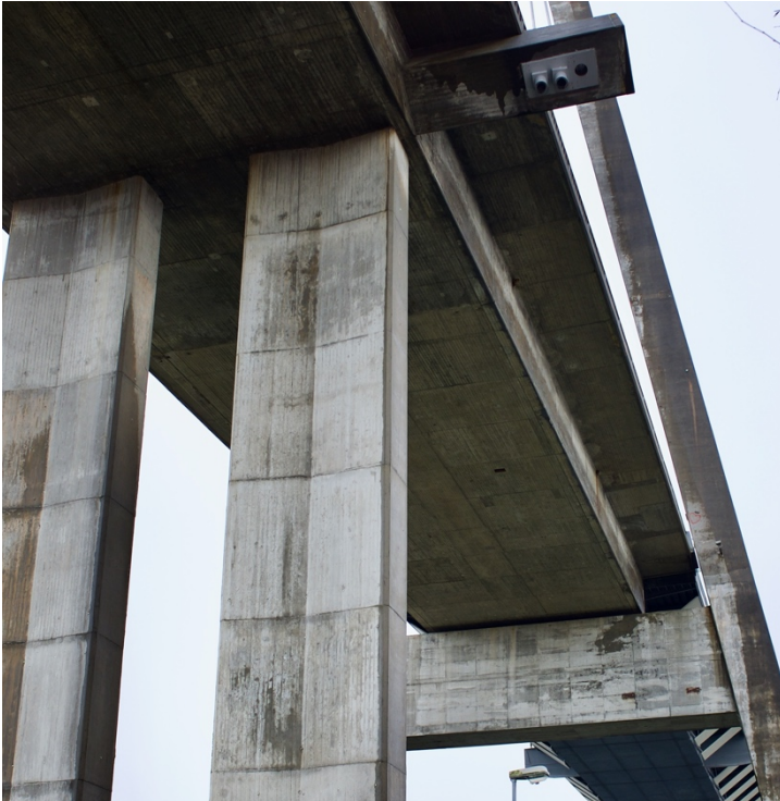
Figure 13: Connection, deck with support pillars and crossbeam
