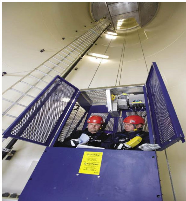
Figure 20: Elevator in the wind turbine (Zipp, 2012)
