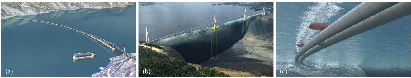
Fig. 3. Concepts for the fjord-crossing project. (a) Curved floating bridge, (b) tension-leg platform supported floating bridge, and (c) submerged floating tunnel.
