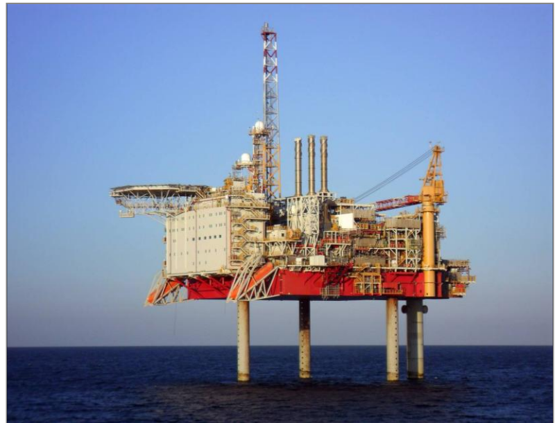
Figure 2-16 Photograph of the Yme platform – a mobile production unit (Holm and Don, 201X).
