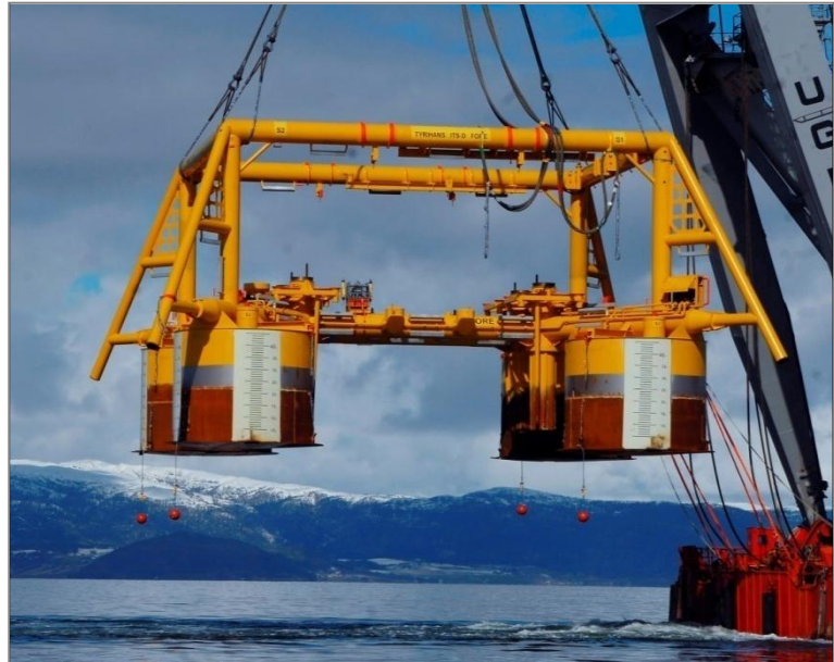
Figure 2-10 Photograph of a subsea template used in the development (Johansen, 2010).
