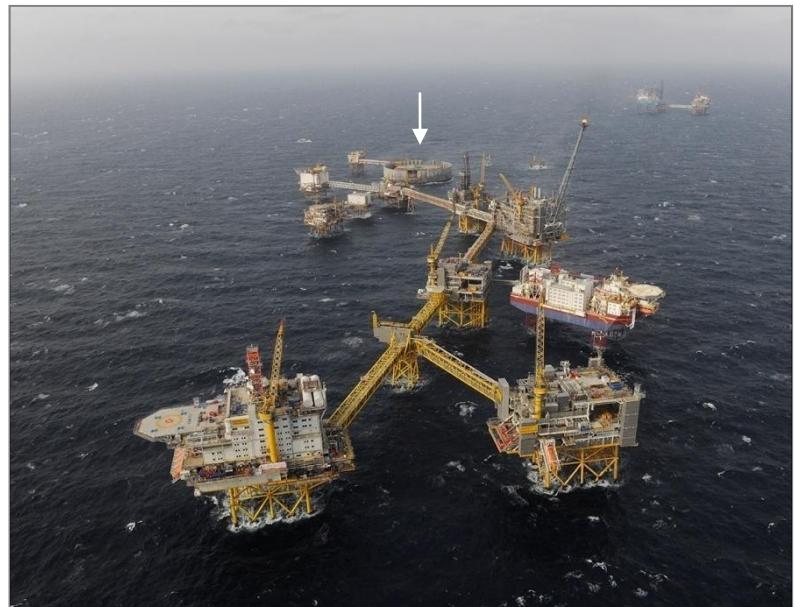
Figure 4-2 Photograph of the Ekofisk complex (Alsvik, 2013). Notice decommissioned oil storage tank in the background.
