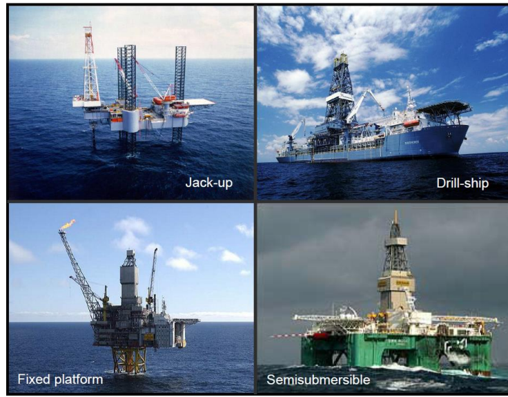
Figure 2.2: Examples of offshore drill rigs [7]
