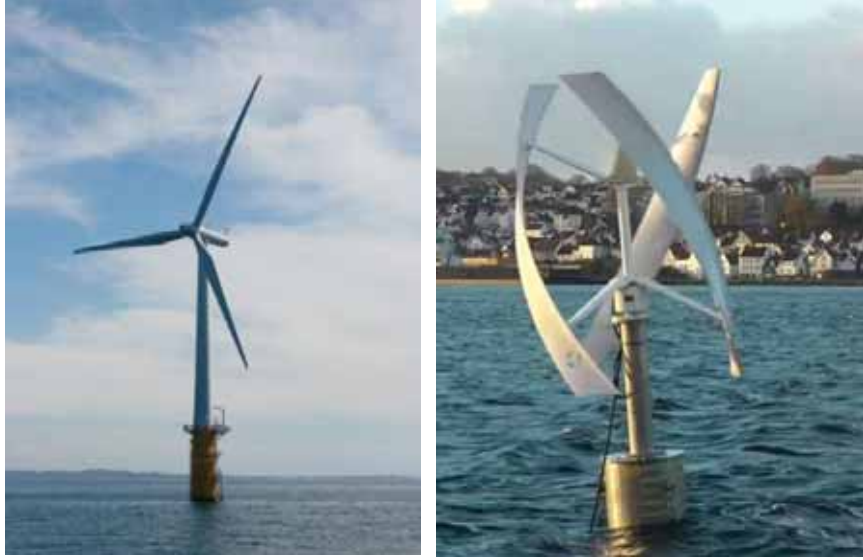
Figure 6: Two floating wind turbine concepts developed in Norway, Statoil's horizontal axis turbine, Hywind, photo: Lene Eliassen (left) and Gwind's vertical axis turbine, Spinwind, photo: Simen Malmin (right).
