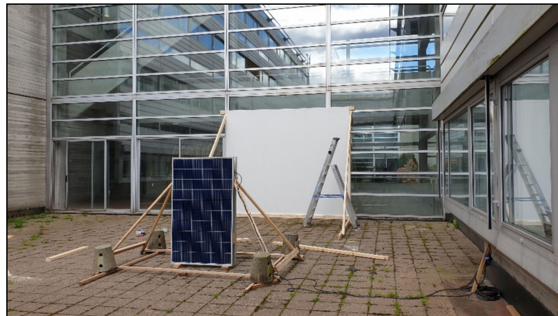
Figure 3. The panel cladding installation phase.
