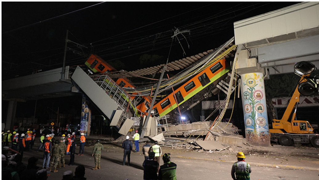
Figur 22: T-banebru kollaps i Mexico City, Mexico [32]
