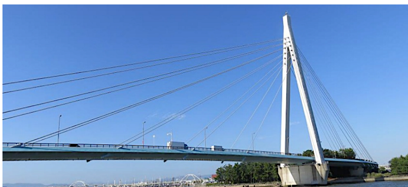
Figur 7: Tsuneyoshi Ohashi bru. Osaka, Japan [4]
