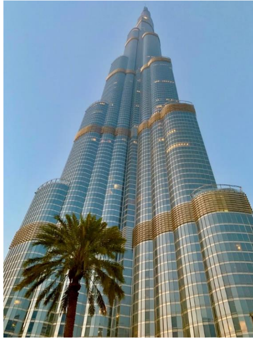
Figure 5.4: Burj Khalifa, located in Dubai is the World's tallest building (828 meters). Built as a Y-shaped structure with setbacks (Photo courtesy of tourist-destinations.net) [57].
