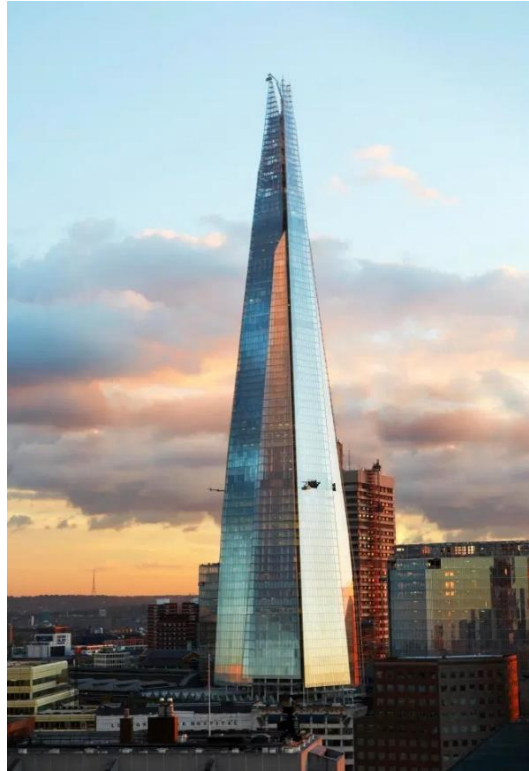
Figure 5.3: The shard in London. Built using the tapering method, influenced by spires of London churches and masts of tall ships from the 1800s. The shard is London’s tallest building, 310 meters high consisting of 95 story’s (Photo courtesy of Getty Images) [55].
