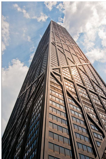
Figure 5.1: John Hancock Center in Chicago, built using the system of framed tubes. The Diagonal bracing is continuous for all faces of the building. The bracing is connected to the columns, forcing loads to transfer from exterior structure to the interior columns (Photo courtesy of Antoine Taveneaux) [37].
