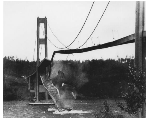
Figure 2.6: Tacoma Narrows Bridge collapsing in 1940, due to oscillation caused by vortex shedding. Only 4 months after opening [9].
