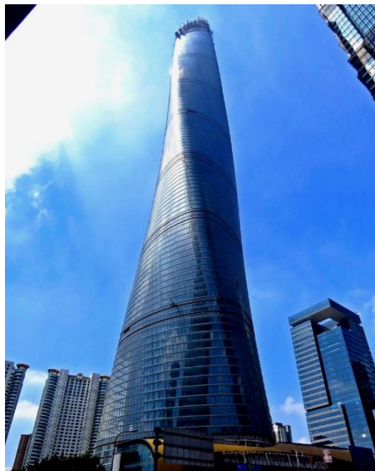
Figure 5.6: Shanghai Tower. World’s second tallest building at 632 meters, and the tallest in China (Photo courtesy of Tansri Muliani).
