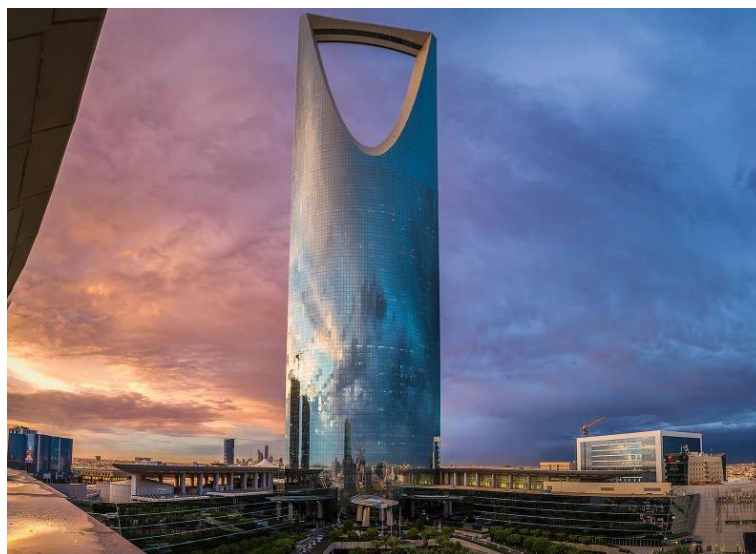
Figure 5.5: Kingdom Centre in Saudi Arabia. The Building is 302 meters high and is connected at the top by a 56 meters bridge with public observation deck, allowing for view over the capital, Riyadh (Photo courtesy of kiwicollection.com) [58].
