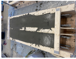
(1) Fresh concrete 35 mm
