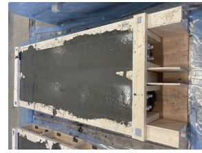
(3) Fresh concrete 85 mm
