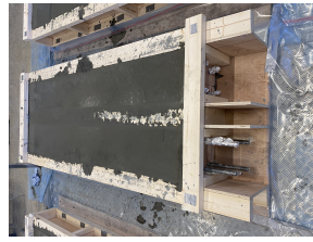
(2) Fresh concrete 60 mm
