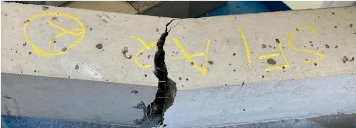
Figure 3-20: Flexural failure of day 28 SFRC specimen
