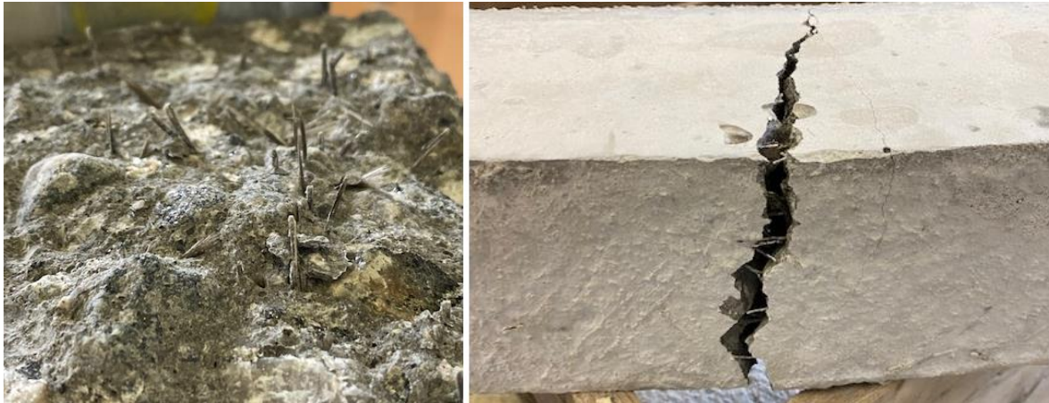
Figure 3-23: Cracked cross section of day 28 BFRC
