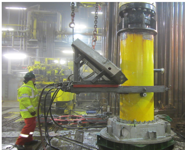
Figure 4.4: Bandsaw cutting operation. (Claxton Engineering, 2020a)
