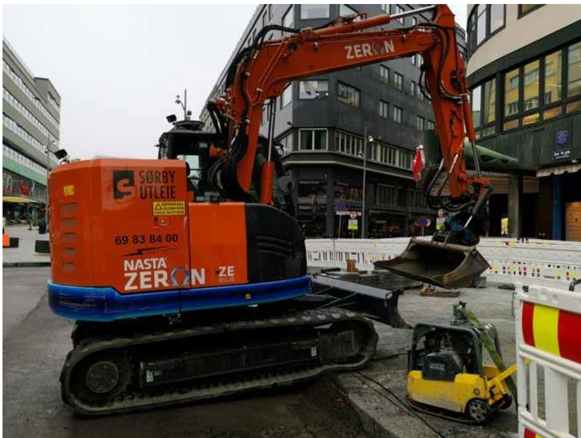
Figure 3. 8-ton electric excavator in Olav Vs gate, Oslo (Bymiljøetaten, 2020, p. 24)
